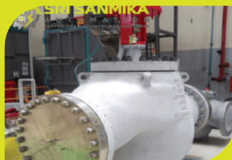
FLANGES FOR VALVE LEAKAGE TESTING PROCESS
